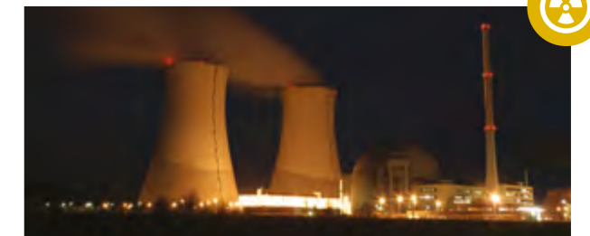
Nuclear Access Control
